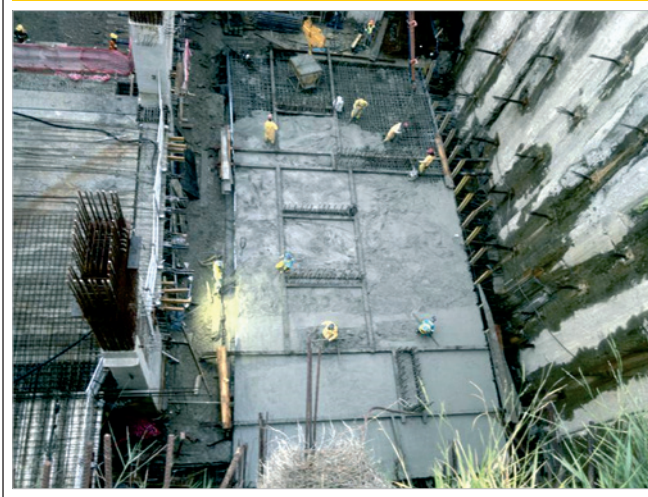
Figure 9 – Finishing the last layer of the footing
