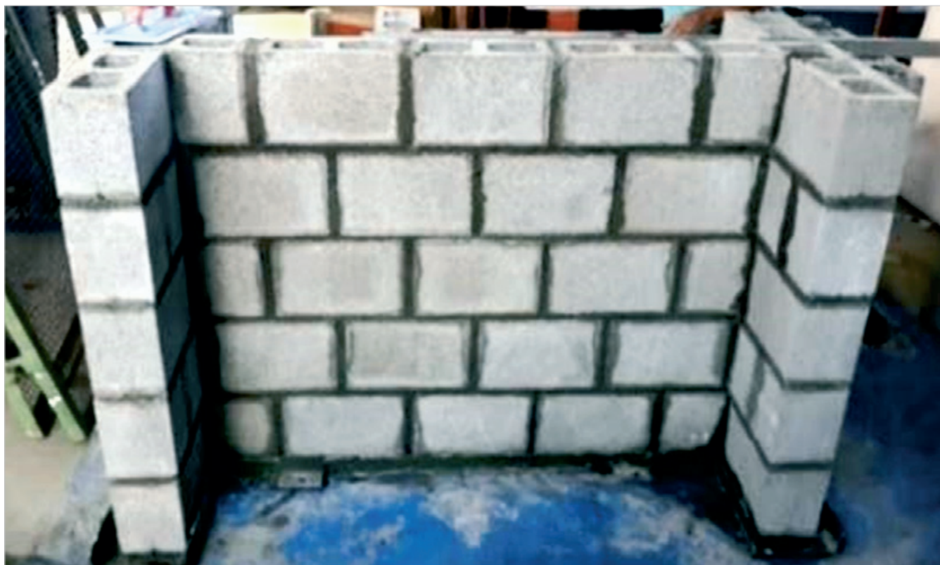
Figure 2 - Executed first step of the flanged wall
