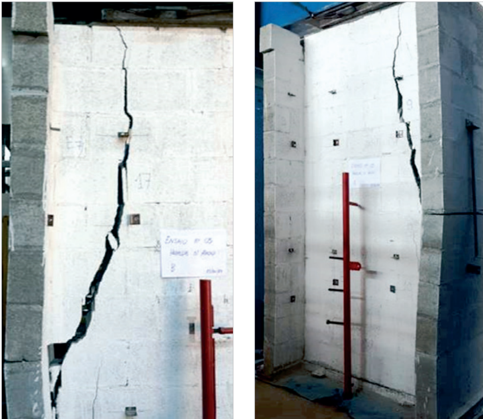
Figure 16 - Failure - flanged wall without central support 05
