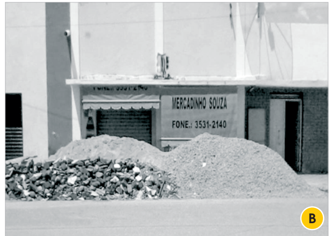
Figure 3 - Layout of materials: a) and d) water tanks, b) materials stored on public streets and close to rubble, c) sand storage
