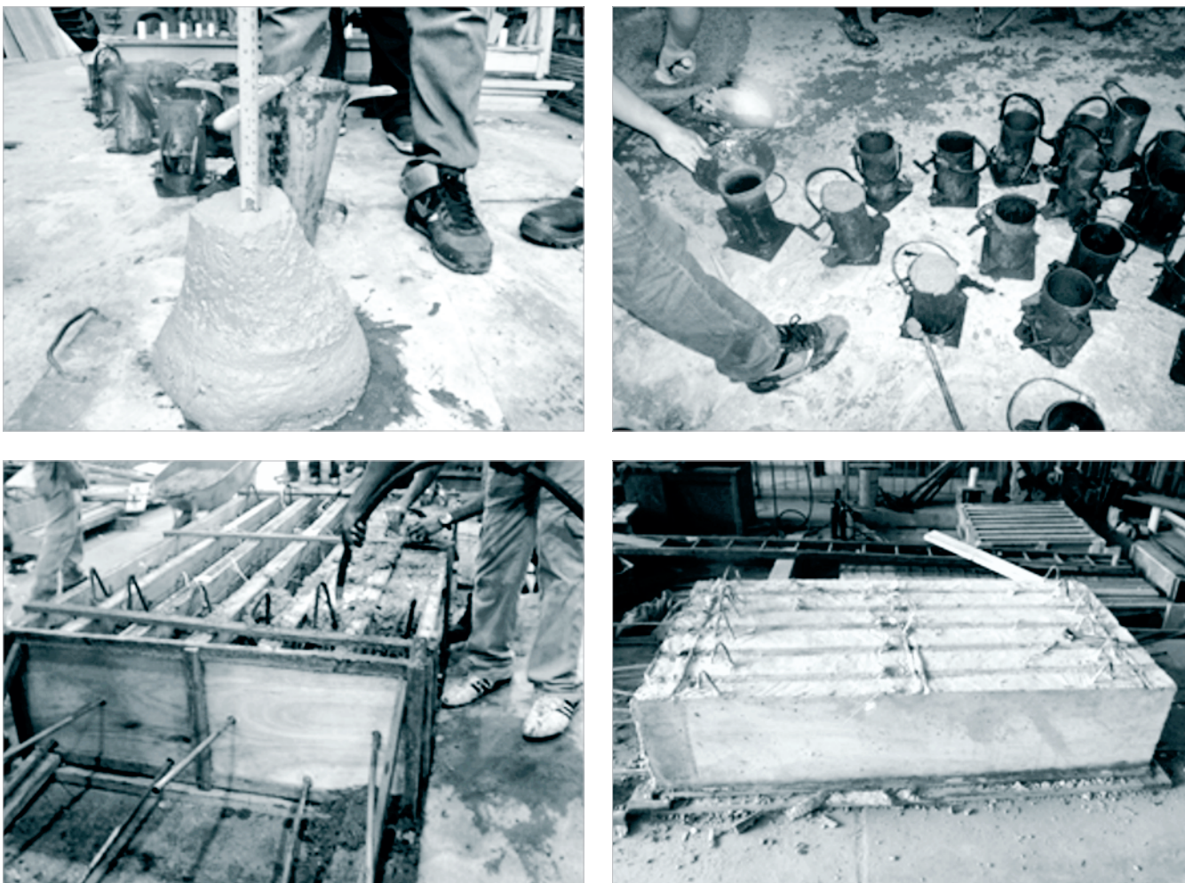
Figure 5 - Beams' executive process
