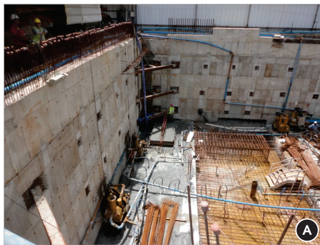
Figure 5 – Detail of concreted phase, joint to the reinforcing wall, with a curing mat over the surface and of curing procedure (mat being soaked)
