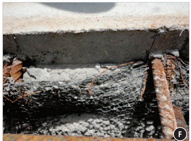
Detail of finishing obtained by upper wooden support barrier, wire mesh just underneath, will yet be cut
