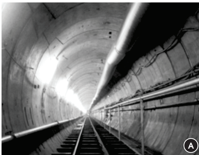
Figure 15 – Built tunnel in Osaka (a) using prestressed and precast concrete segments (b), (22)
