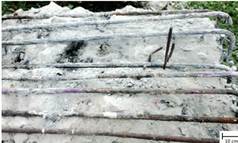
Figure 4 Full exposition of the foundation block protruding reinforcing steel
