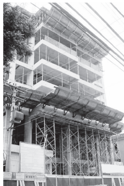
Figure 4 Construction aspect at the second construction stage
