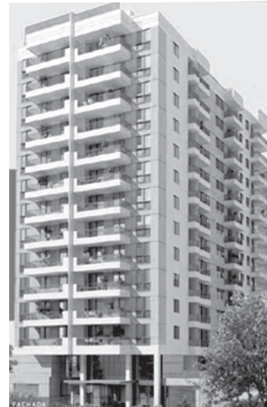
Figure 1 Building frontal view
