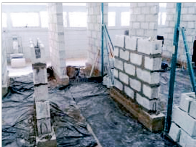
Figure 11 Wall with mid-height bond beam
