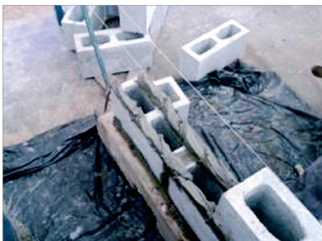
Figure 13 Face-shell bed mortar joint wall construction
