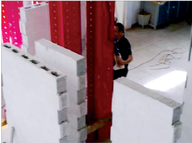
Figure 15 Walls capped with mortar
