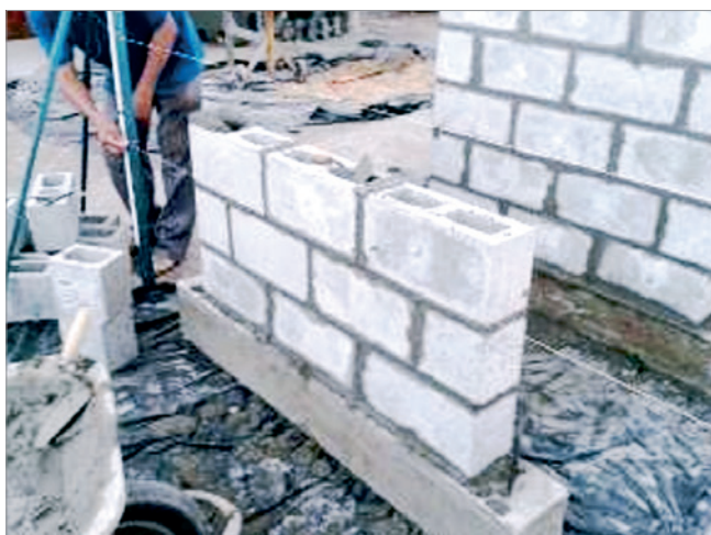
Figure 9 Hollow wall construction
