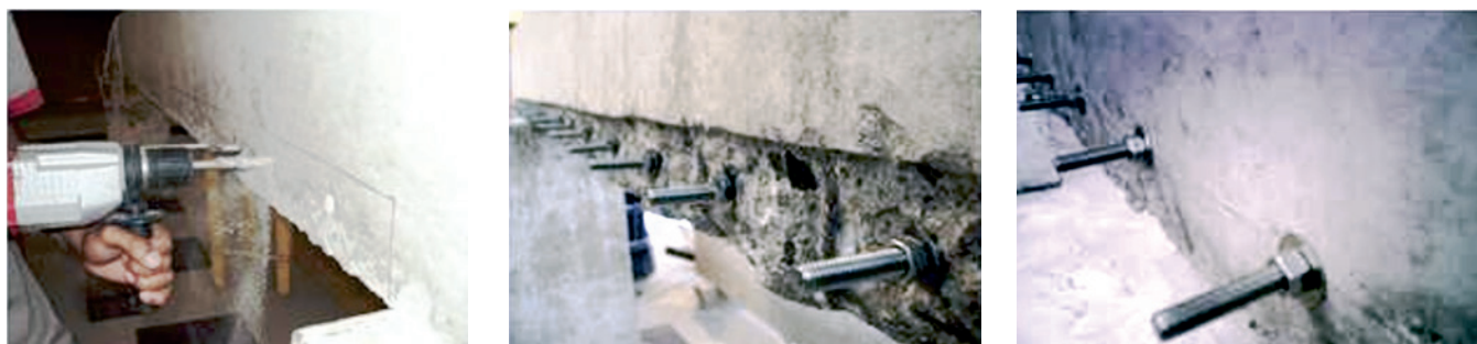
Figure 2 Expansion bolts
