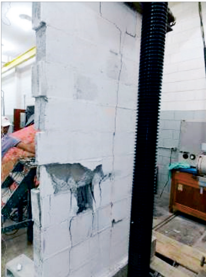
Figure 29 Wall vertical cracking and failure
