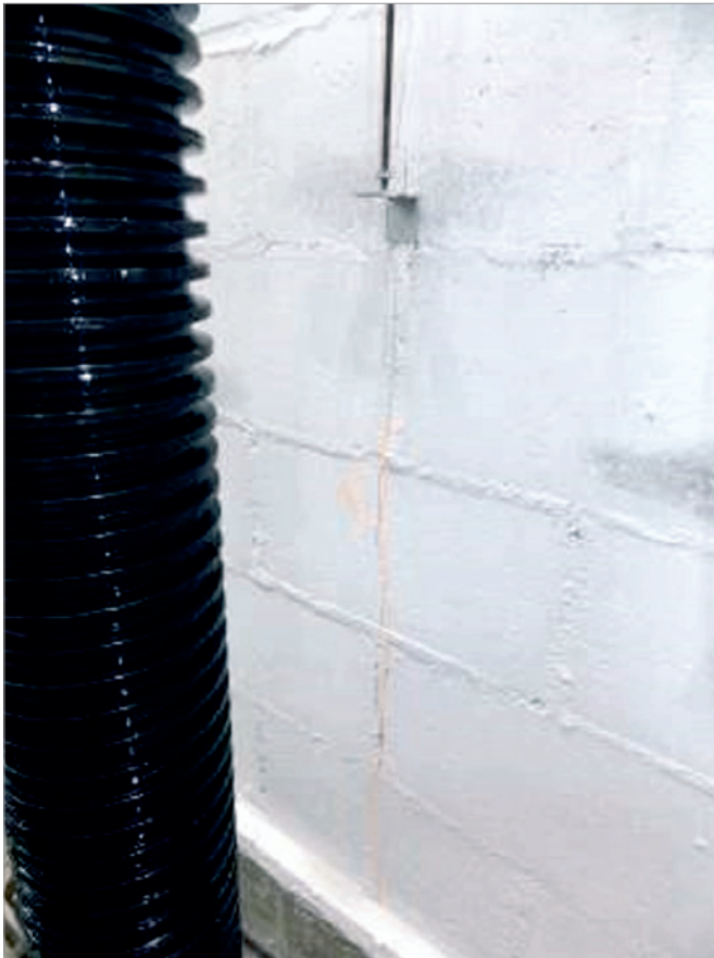
Figure 31 Grouted wall failure
