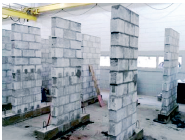
Figure 2 Wall before testing
