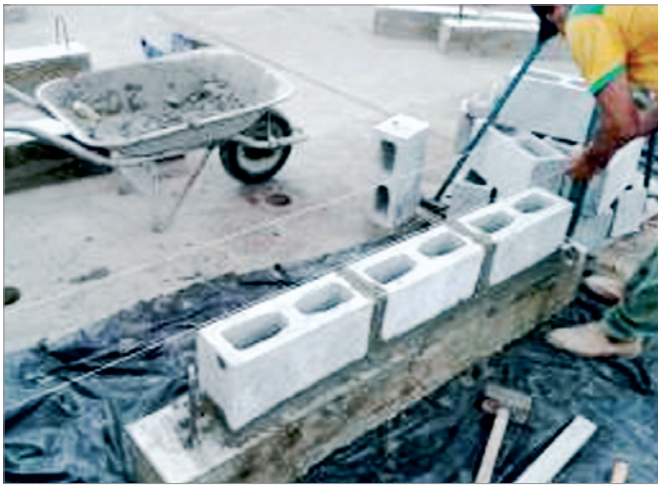
Figure 7 Corner gauge to aid wall construction
