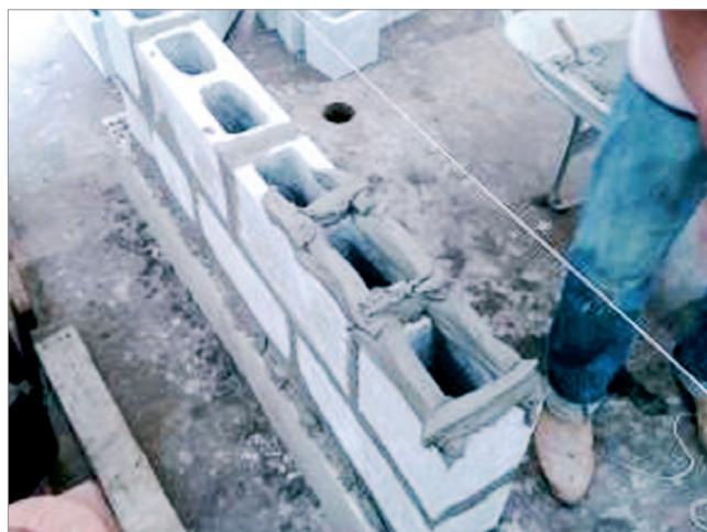
Figure 12 Full bed mortar joint wall construction
