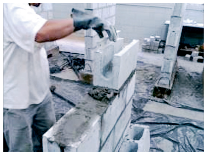
Figure 10 Mid-height bond beam laying
