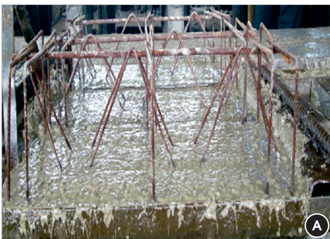
Concreting of the upper side of the panel
