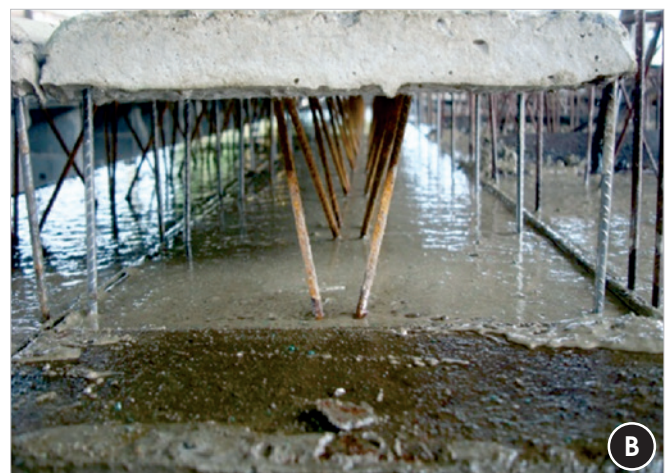
Concreting of the opposite side
