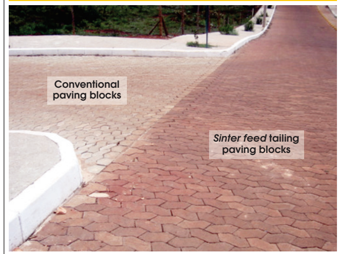
Figure 11 – View of an experimental section of pavement showing conventional concrete blocks and blocks containing sinter feed tailings
