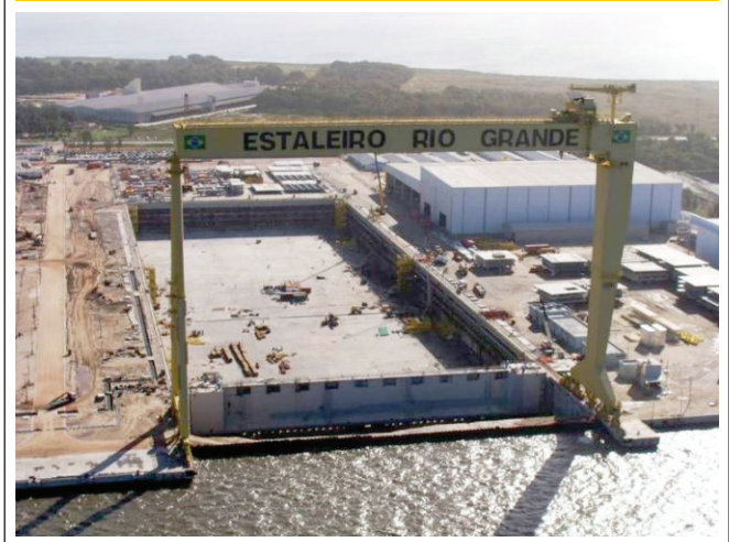
Figura 3 – Aerial view of the Rio Grande dry dock yard - ERG1
