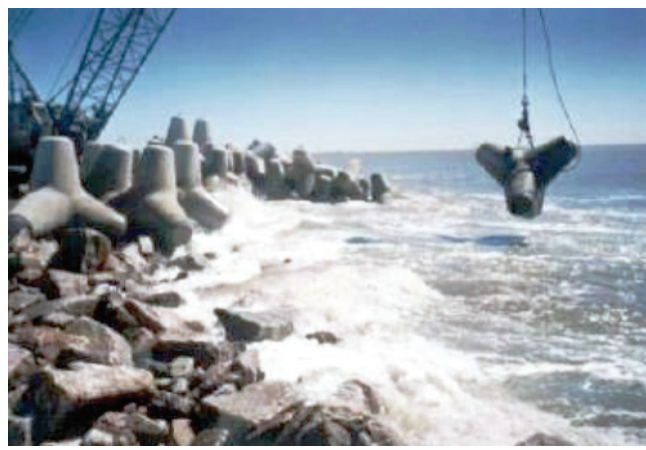
Figure 1 – Installation of the tetrapods in the construction site of Barra do Rio Grande breakwaters expansion project (Source: Migliorini, 2011)
