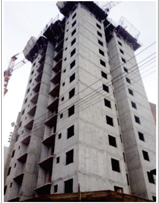
Figure 1 – Building Condomínio das Árvores under construction – 13 type floors concreted
