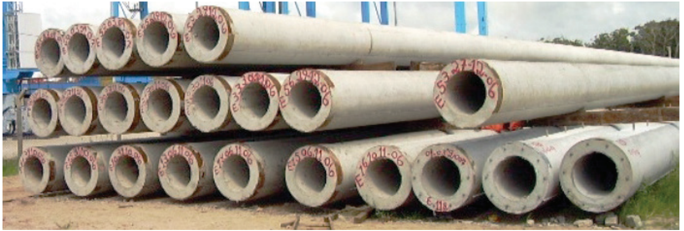
Figure 2 – Piles of the pier (Source: FURG)
