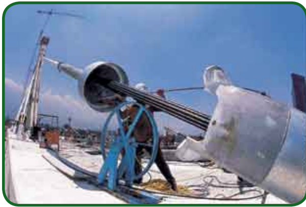
Fig. 16 – Strand by strand installation
