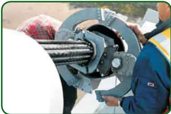
Fig. 14 – Dismantling of the friction damper
