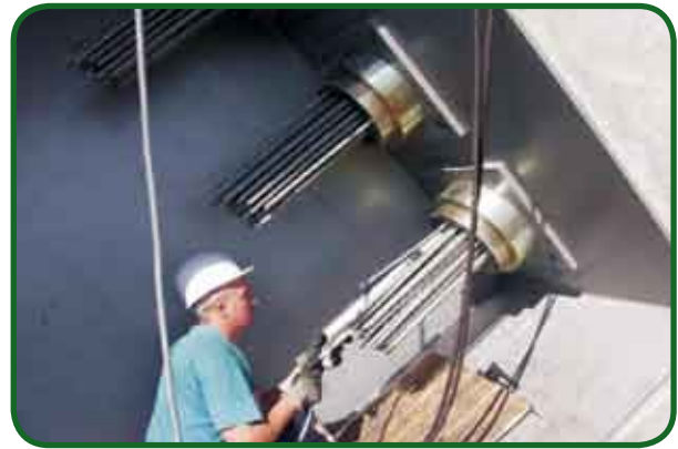
Fig. 17 – Stressing operation with the automatic monostrand stressing system
