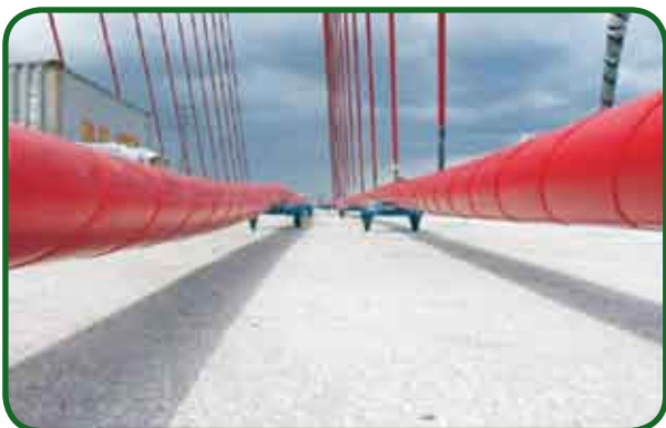
Fig. 6 – Stay pipe with helical ribs
