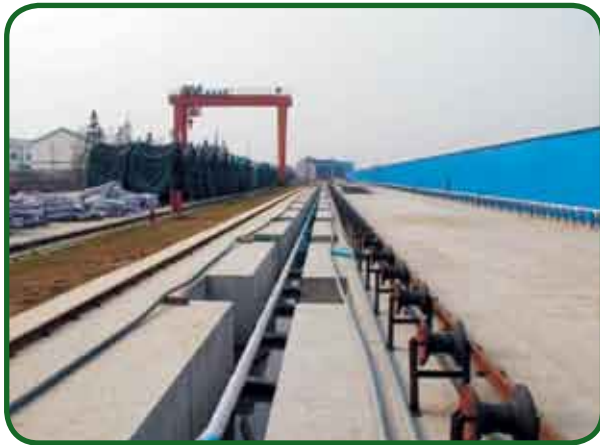
Fig. 11 – View of the 216 m long parallel wire cable
