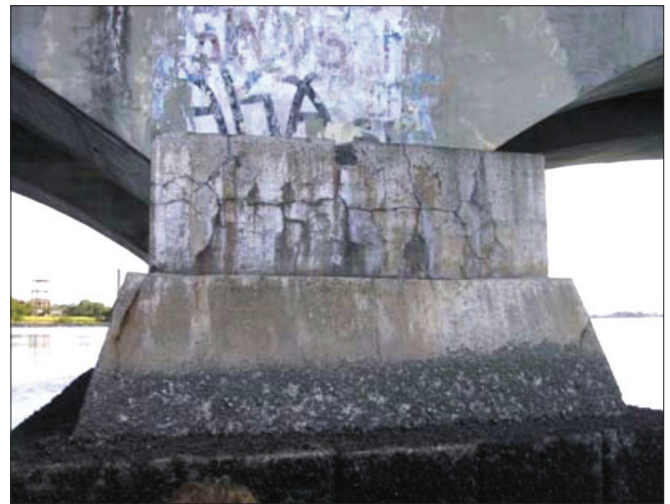
Figure 1 – PGB view, emphasizing some deteriorated parts
