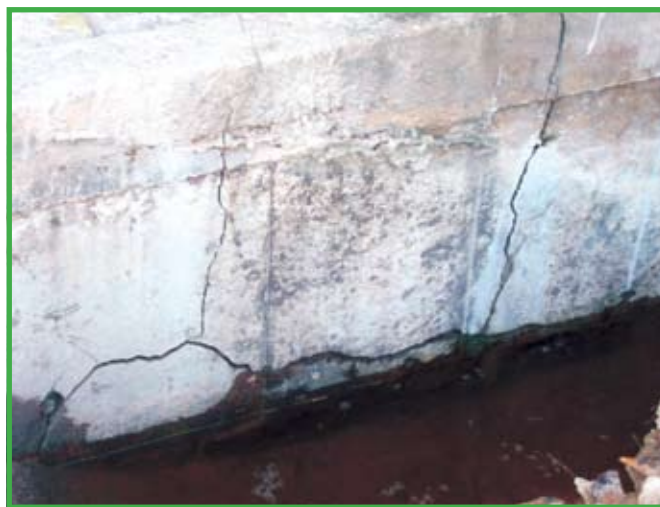
Figure 10 - Detail of the cracks on the side of the block
