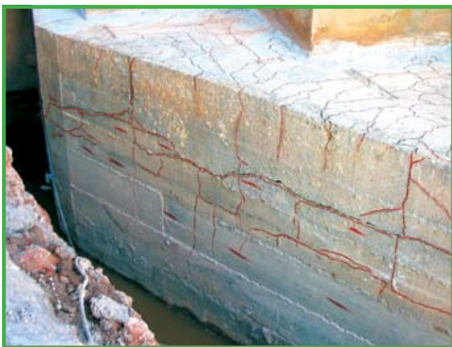
Figure 15 - Intense cracking on one of the blocks, with greater occurrence on the top and sides, down a certain length along the side, where the reinforcement is less intense
