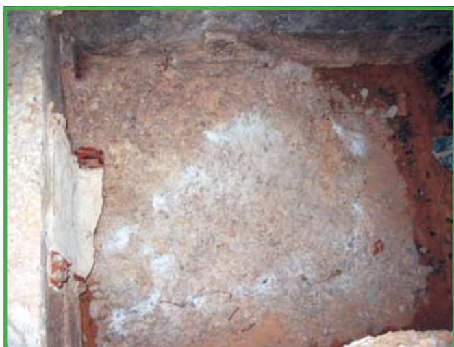
Figure 4 - Concentric cracking in one of the base plates in the building close to the Areia Branca Building, where the holes bored for epoxy injecting can be seen
