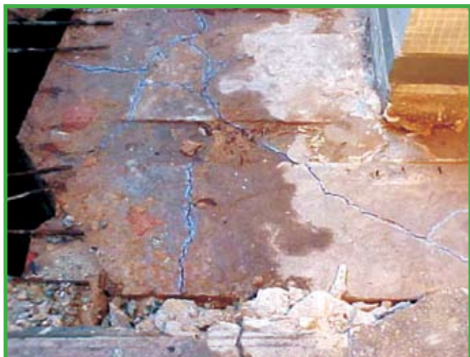
Figure 12 - Random cracking on the top side of the block
