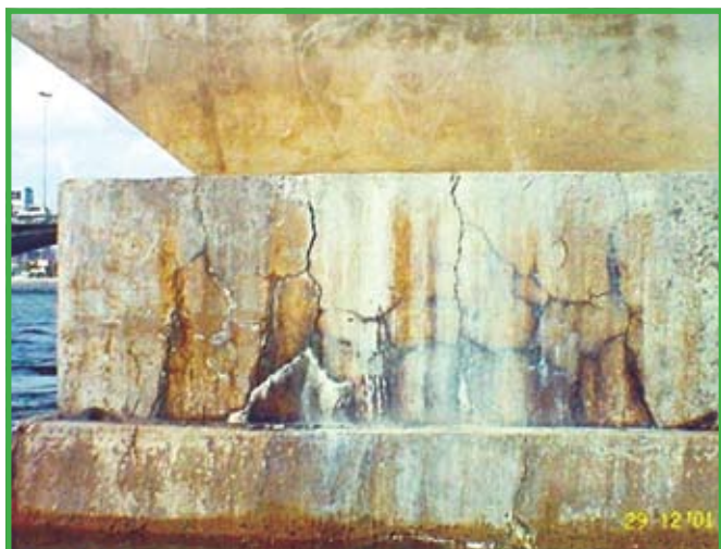
Figure 3 - Fissures and crackings that are typical of expansion induced by the alkali-aggregate reaction in one of the blocks of the Paulo Guerra Bridge
