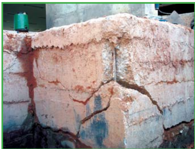
Figure 17 - Detail of a crack on one of the corners of the block
