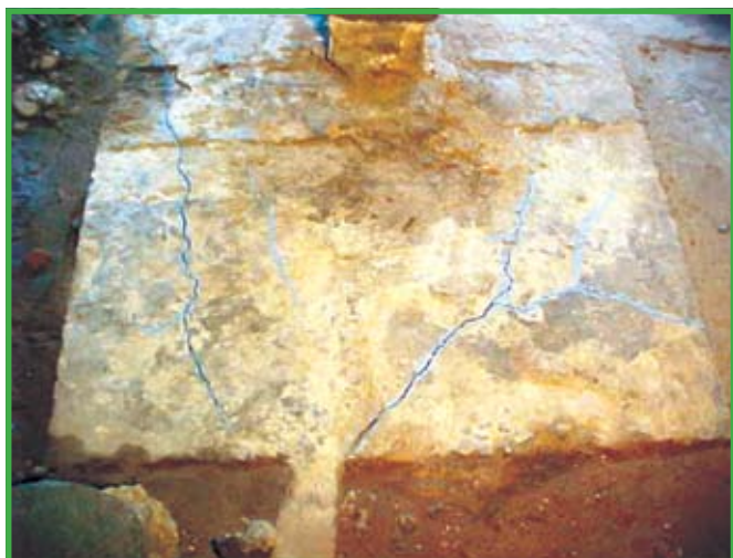
Figure 11 - Detail of a block in which the tie restricted the expansion towards it, thus inducing wedge-shaped cracking
