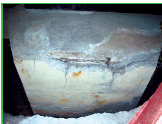
Figure 6 - Foundation block where cracking was first detected due to the appearance of vertical cracks that led to the excavation down to the foundation block
