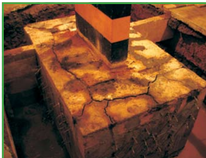
Figure 5 - Foundation block with top surface seriously cracked, featuring openings of up to 25 mm in some areas
