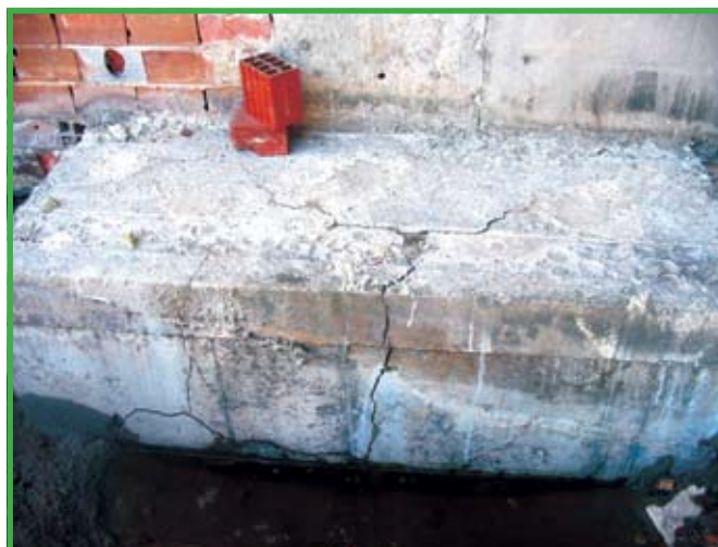
Figure 9 - Cracks on the top side of the blocks, descending to the sides
