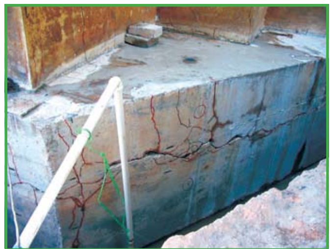
Figure 16 - Horizontal crack with a wide opening on the side of one of the blocks. In that area, there is a 35 cm zone without vertical reinforcement, which could restrict the expansion in that direction
