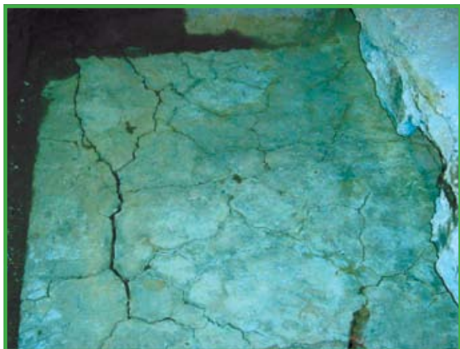
Figure 8 - Detail of crack on the left side of another block, with an opening of more than 30mm
