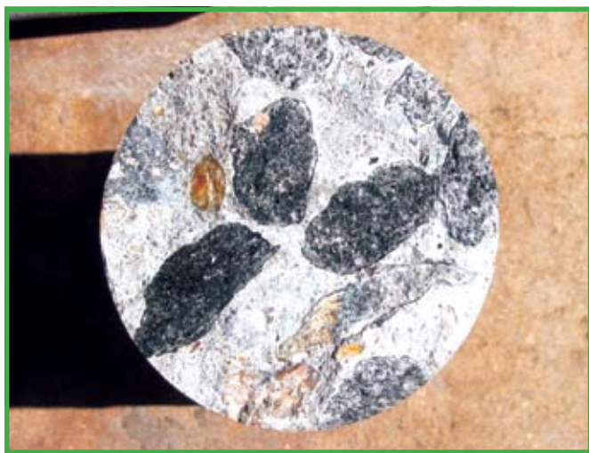
Figure 1 - Cracked side of the core
