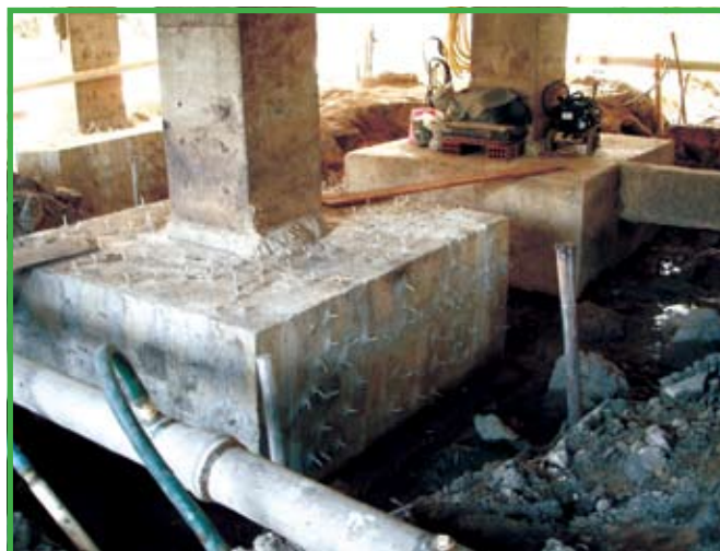
Figure 20 - View of two rectangular blocks, the first being intensely cracked, while the second (behind) has no cracking symptoms
