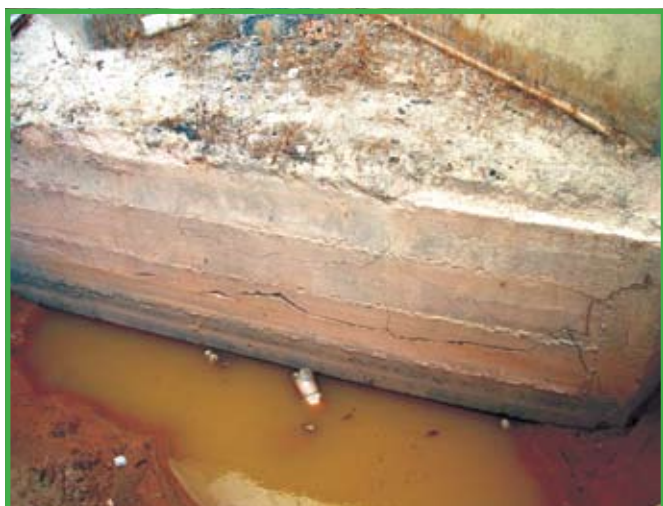
Figure 18 - Side view of one of the cracked blocks
