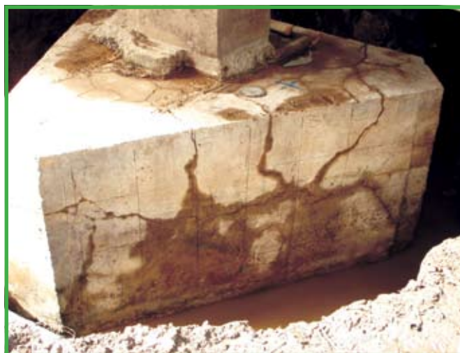
Figure 19 - View of a cracked triangular block
