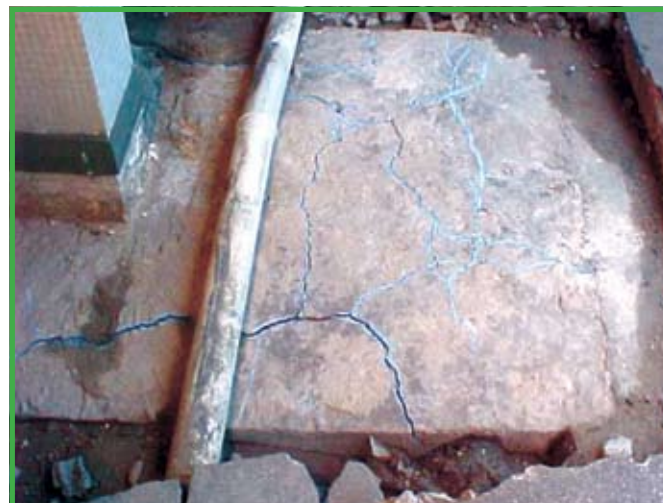
Figure 13 - Random cracking on the top side of the block
