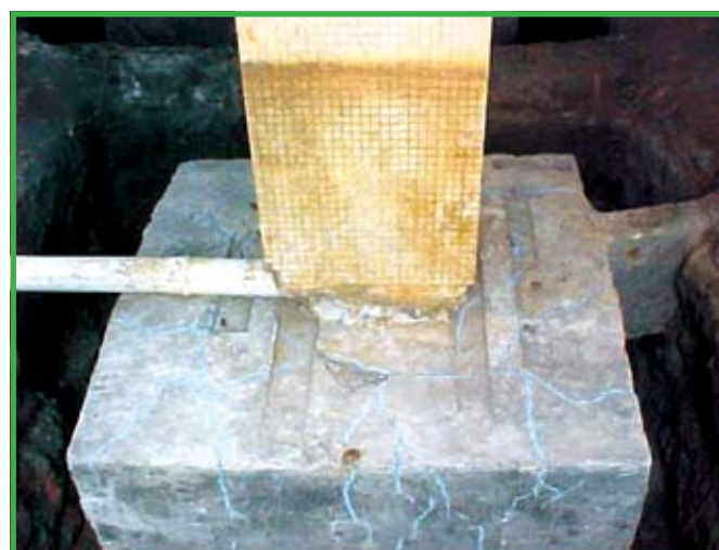
Figure 14 - Random cracking on the top side of the block, descending along the vertical side
