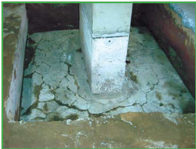
Figure 7 - Intense cracking on one of the foundation blocks in the downtown commercial building
