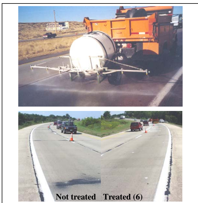
Figure 3 - (A). Topical application of lithium-based solutions at the surface of a pavement section affected by ASR (B). Condition of not-treated (control) and treated sections (after six topical treatments with lithium nitrate solution) of concrete pavement affected by ASR in Delaware (USA). Spalling of concrete at joints is more frequently observed in the untreated sections (Pictures A & B: courtesy of D.B. Stokes, FMC Corporation – Lithium Division, Charlotte, USA).
