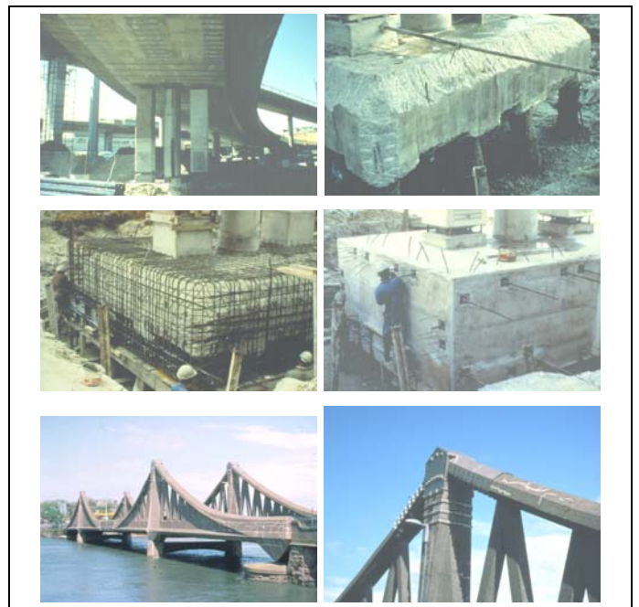
Figure 5 - (A-D). Highway structure affected by ASR in South Africa. (B). The cracked concrete in the pile caps was first removed. (C). Additional steel reinforcement was added around the pile cap. (D). External strengthening is provided by means of prestressed cables. (E). General view of Montrose bridge (Scotland) (F). The strengthening remedial work consisted in reinforcement by straps, plates and tensioned bolts to provide full containment for the top chord and tower top area. (A to D: courtesy of R.E. Oberholster, PPC Technical Services, Cleveland, South Africa) (E and F: courtesy of J.G.M. Wood, Structural Studies & Design Ltd., Chiddingfold, UK).
