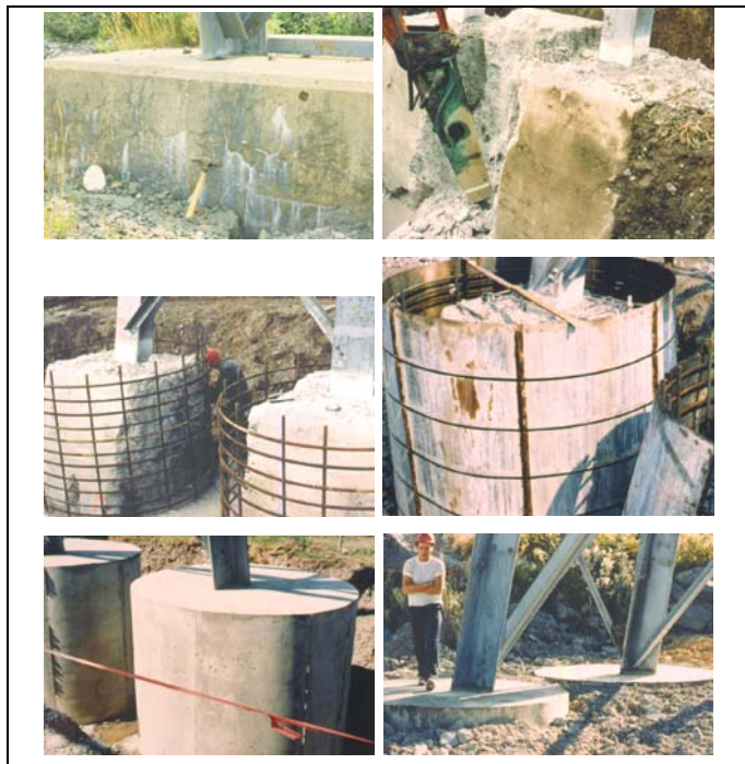
Figure 6 - (A to F). Repair of a group of electricity tower concrete foundation affected by ASR in Quebec City (Canada). (A). Map-cracking and gel exudation affecting a 29-year-old concrete foundation. (B). Splitting the foundations in two blocks. (C to F). Encapsulation with reinforcing steel and silica-fume concrete.
