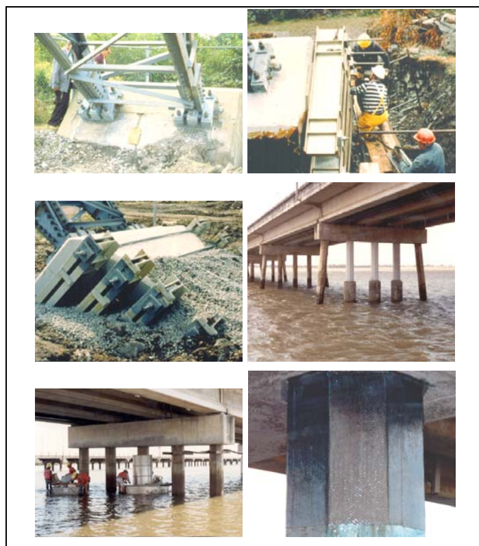
Figure 7 (A) - Concrete anchor block for electricity towers affected by ASR (B and C). External strengthening using steel frames, rods and plates. (D to F). Bridge structure affected by ASR in Australia. (D). Glass-fibre composite repair to 500 above high water level and concrete encasement to bed level. (E). View of cofferdam and split aluminium formwork. (F). Wrapping with two layers of carbon fibre composite materials. (Pictures D to F: courtesy of A. Carse, Queensland Transport, Brisbane, Australia).
