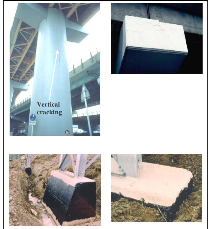
Figure 2 - (A). Reinforced concrete pier of the Hanshin expressway in Kobe (Japan) affected by ASR. Vertical cracks reappearing a few years after the treatment with various types of coating. (B). Beams were also repaired by using either polyurethane resins or epoxy resins; cracks also reappeared shortly after the treatment. (C & D). Massive electric tower foundations affected by ASR. Some of the foundations were treated by applying a bituminous coating on the buried surfaces and a flexible water-resistance polymer membrane on exposed concrete surfaces.
