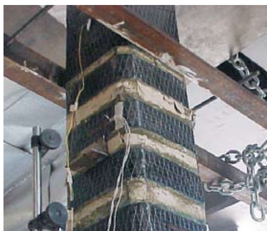
Figure 6 – Rupture of the concrete between the straps
