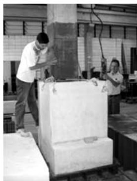
7 th ) Raising and temporary fixation of column on socket base
