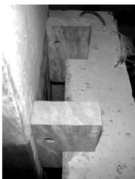
9 th ) Joining of column
