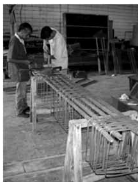
3 rd ) Assembly of column reinforcement
