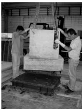
5 th ) Raising of socket base for transition piece
