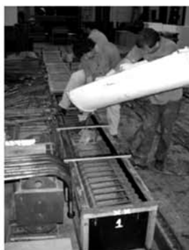
4 th ) Casting of column
