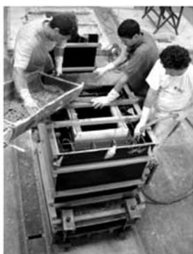
2 nd ) Casting of socket base
