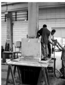
10 th ) Casting of connection joint of elements
