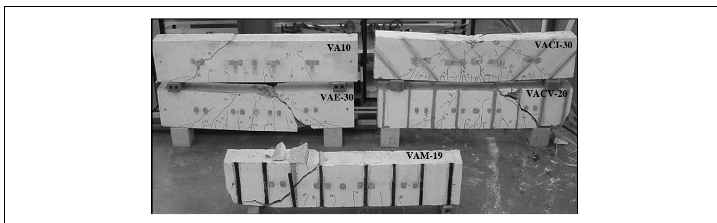
Figure 8 - Failure modes of the beams of A series with 4φ10.
