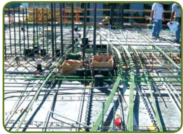
Figure 4 – Alignment of Post-Tensioning Tendons around Openings
