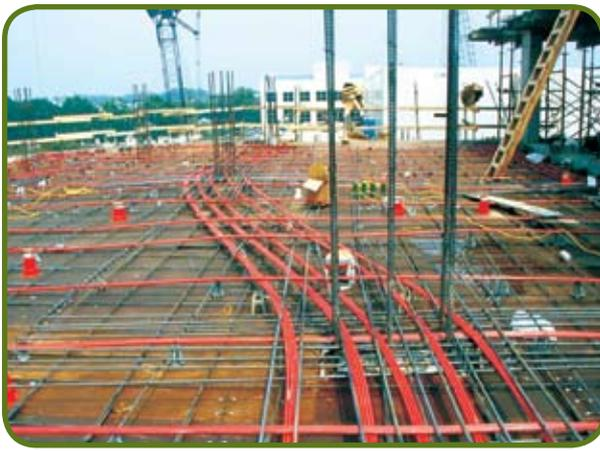
Figure 3 – Flexibility in the Layout of Tendons in a 2-Way Post-Tensioned Slab
