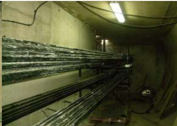
Execution of external prestressing inside the box-girder
