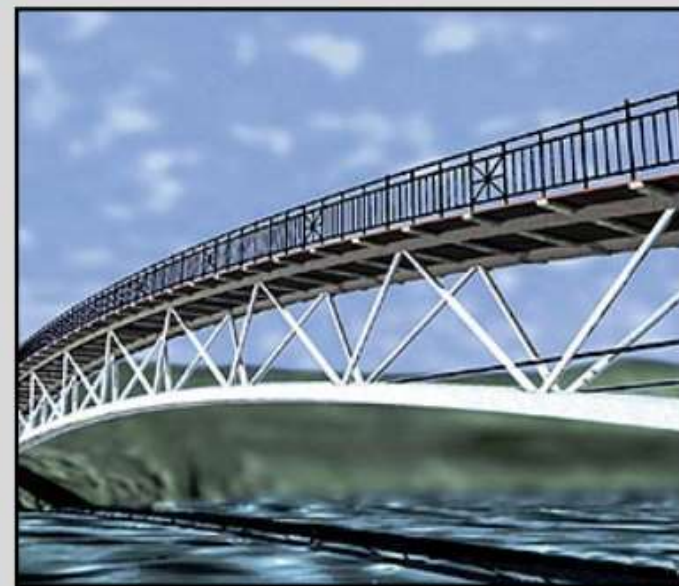
first footbridge made of RPC in Sherbrooke, Canada, 1997
