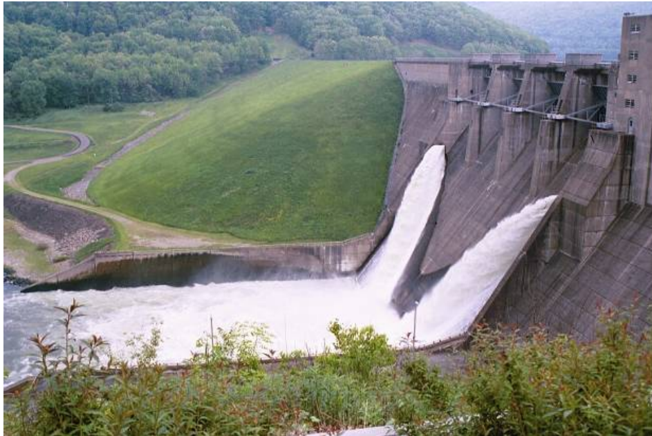
Kinzua dam Stilling Basin, NY Stilling basin repair Still in good shape after 24 years
